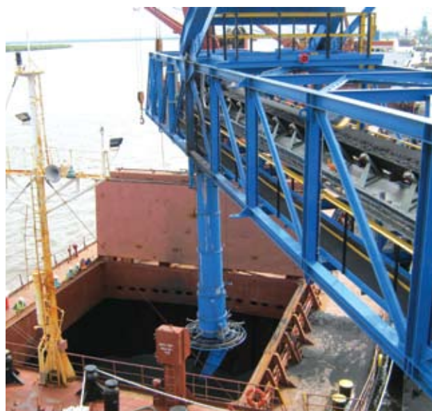
Shiploader loading a vessel at the Grindrod Matola coal terminal, Mozambique.
