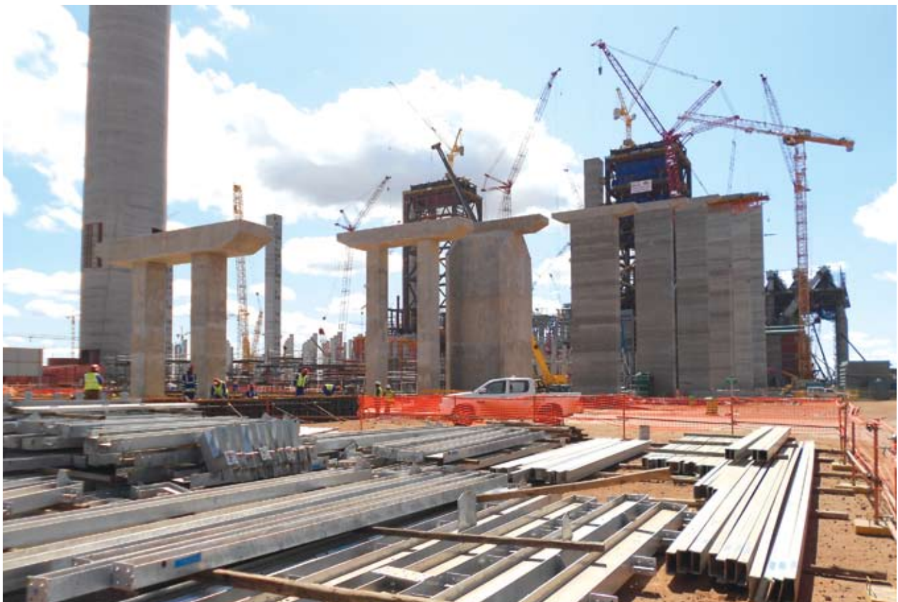
Incline conveyor drive house foundations and steel awaiting erection at Medupi.
