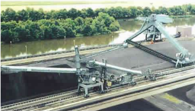
Coaling installation done in Germany, consisting of a slewing and luffing stacker in strata stacking mode with portal scraper re-claimer.
