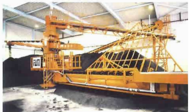
Circular covered stockpile featuring stacker and bridge re-claimer with harrow rake.
